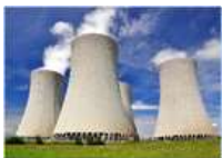
COOLING TOWER WATER
